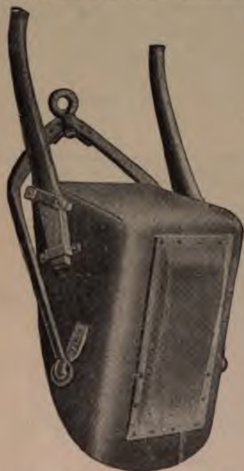
Rear View of Drag Scraper with Double Bottom.
